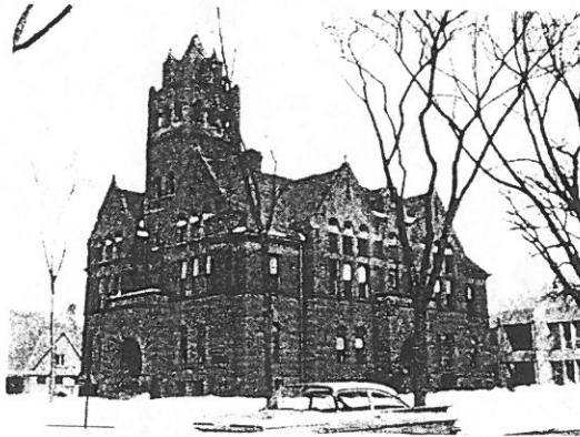
Second Court House, dedicated 1900; still in use.
